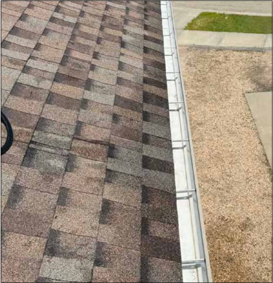
Before and after: Cleaning out eavestroughs is one of the fall maintenance jobs that can help prepare a home for the winter months. Removing leaves and debris allows water to drain properly and helps prevent potential problems when snow and ice arrive.
