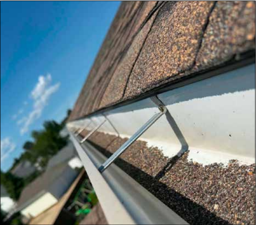
Before and after: Cleaning out eavestroughs is one of the fall maintenance jobs that can help prepare a home for the winter months. Removing leaves and debris allows water to drain properly and helps prevent potential problems when snow and ice arrive.
