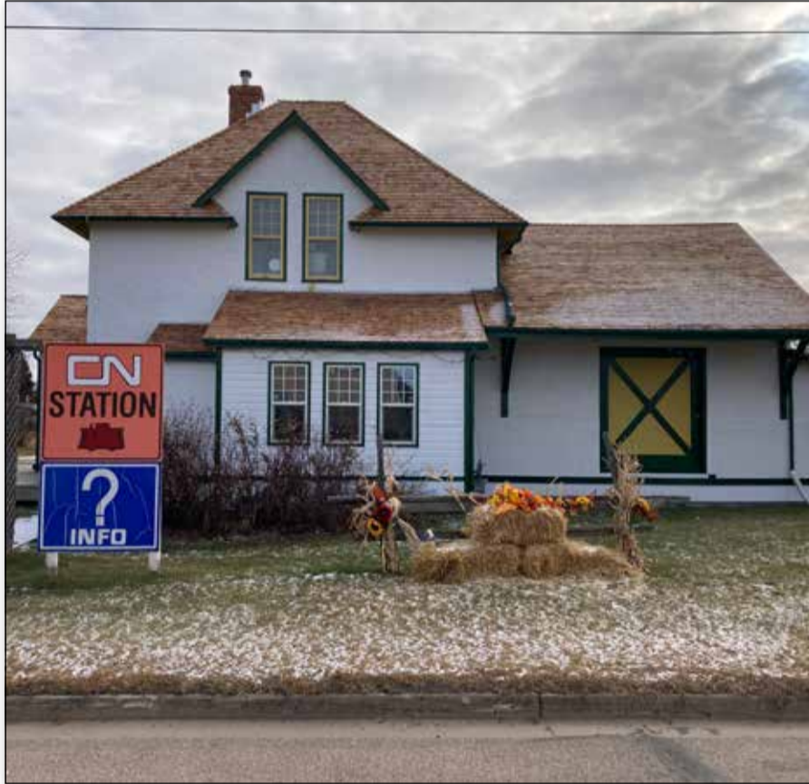
The CN Station in Smoky Lake is an attractive stop for visitors, particularly after the makeover with a new roof and new paint.
