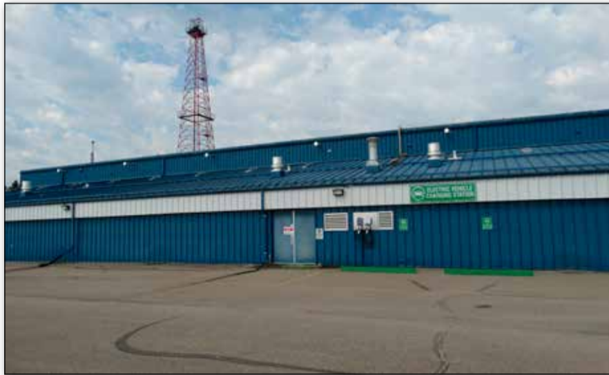
The Town of Redwater has installed two level two EV charging stations at Pembina Place. Photo by Falon Fayant
