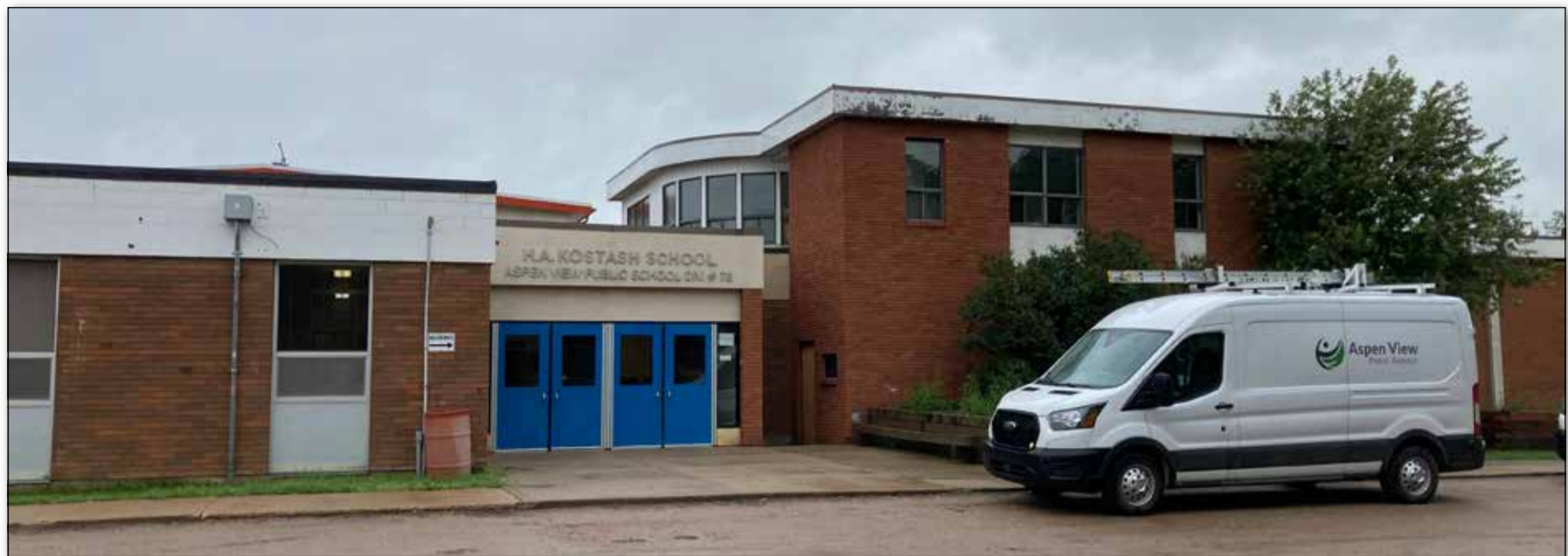
The main building of the old H.A.Kostash school. Smoky Lake lobbied hard for a new school, which was just completed. Aspen View School Division insists on demolition of the entire old school on August 1st.
