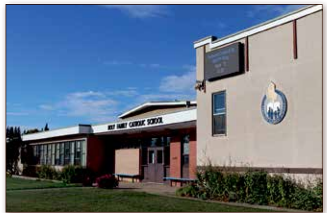
Holy Family Catholic School has been listed among those to receive new buildings in the 2023 provincial budget.
