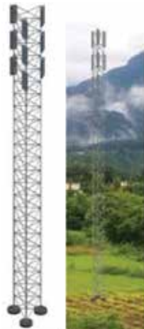
Sample Photo of Existing Rogers Facility (Lattice Tripole Tower): Photo depicts existing facility with top mounted cellular antennas (pin wheel array), microwave transmission dishes, radio equipment, shelter and access road. Illustration only.
