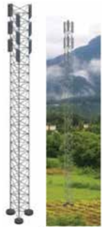
Sample Photo of Existing Rogers Facility (Lattice Tripole Tower): Photo depicts existing facility with top mounted cellular antennas (pin wheel array), microwave transmission dishes, radio equipment, shelter and access road. Illustration only.
