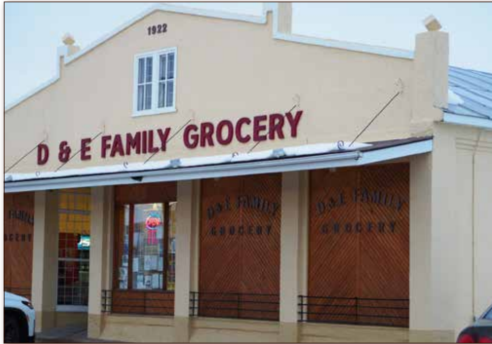
The D&E Family Grocery stands on the main street in the Village of Vilna, and is where the McConnells served the community for over 39 years.
