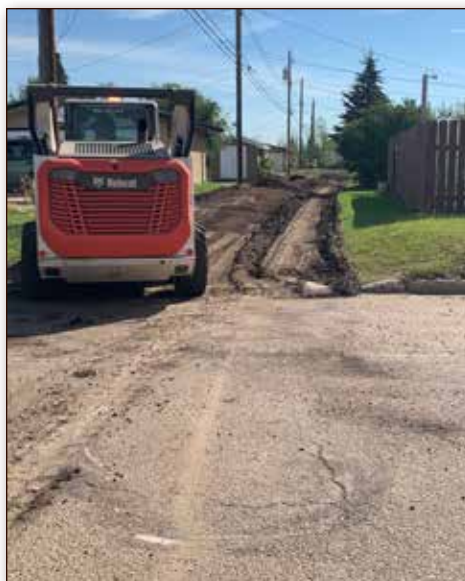
The Town of Redwater has been fixing the back alley between 46 and 47 Street. Staff is laying down recycled asphalt in order to improve parking and alley maintenance for residents. Thank you for your patience as we work to improve our community!
