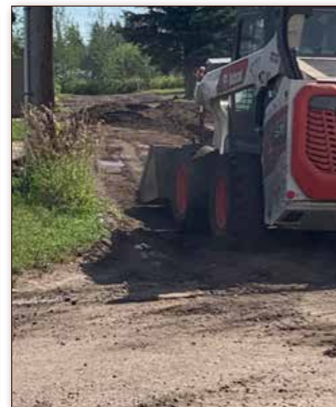
The Town of Redwater has been fixing the back alley between 46 and 47 Street. Staff is laying down recycled asphalt in order to improve parking and alley maintenance for residents. Thank you for your patience as we work to improve our community!
