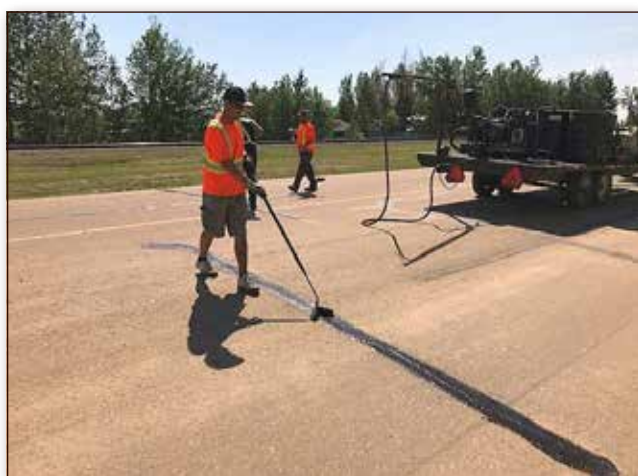
Every year Redwater Public Works completes this project as a key strategy for street preventative maintenance ensuring valuable infrastructure is maintained, keeping the Town moving safely. Crack sealing is the process of placing an adhesive sealant into cracks on the pavement surface, preventing the infiltration of moisture and non-compressible materials into the pavement.
