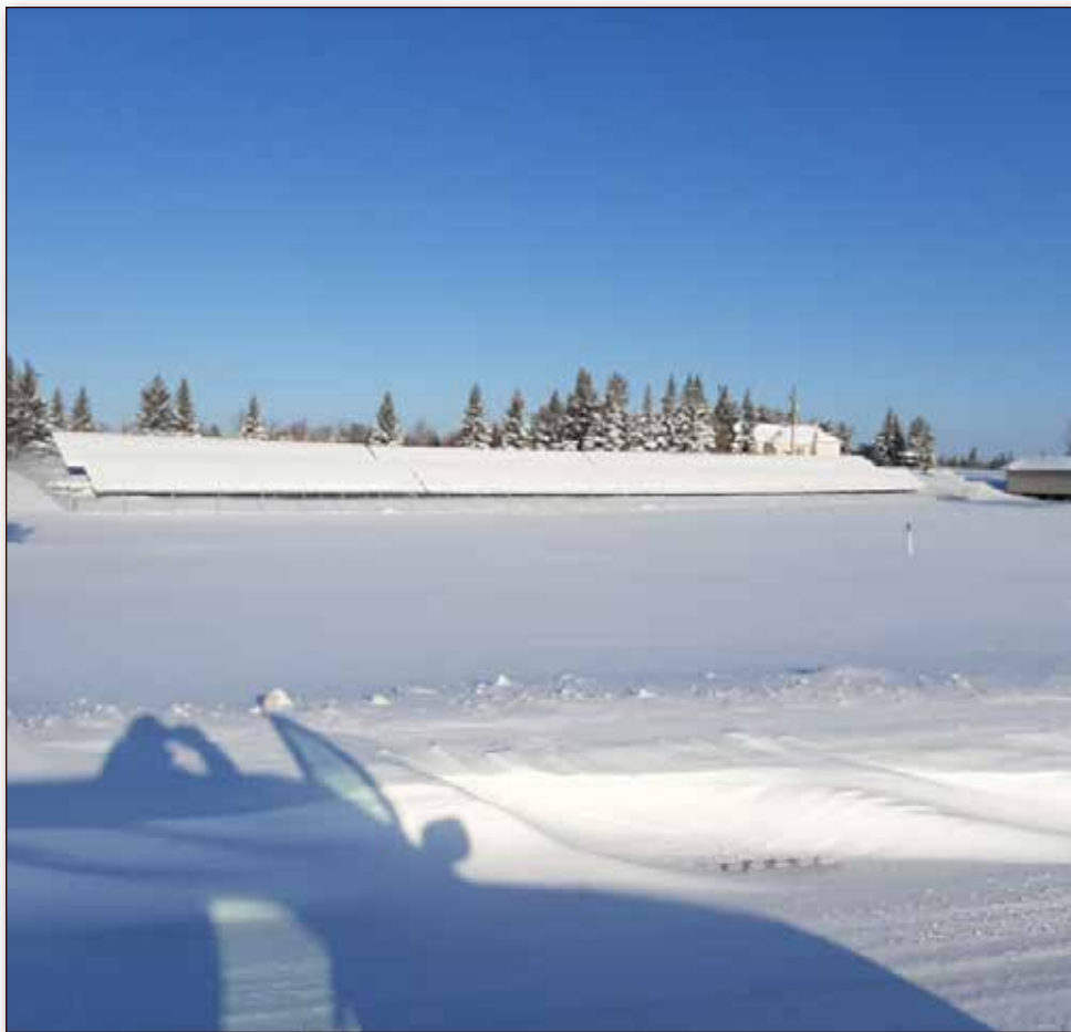
Snow coverage on solar panels only reduces their effectiveness by three percent, as a NAIT study shows.
